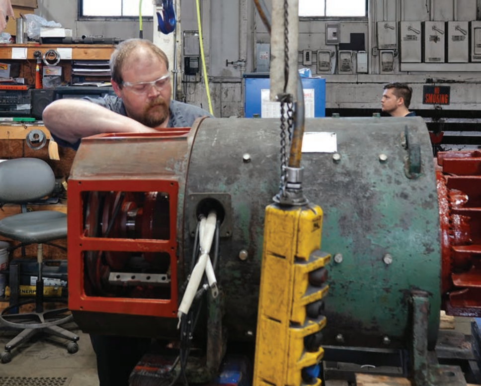
At EMT's St. Bernard shop, Brad Hartman works on a d-c motor for an extruder application.
